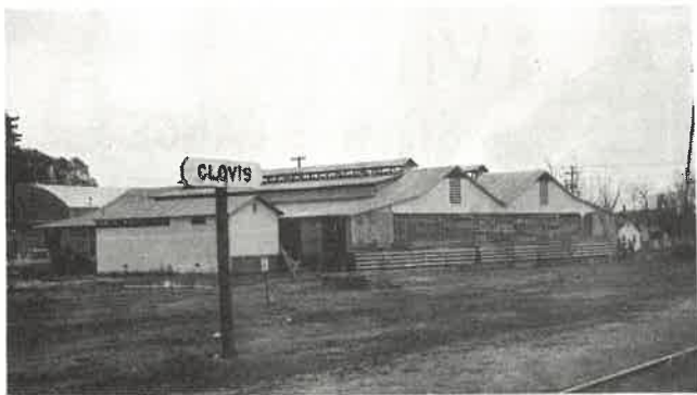
ORIGINAL UNUSED PACKING SHED
